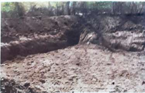
Excavation of farm pond
